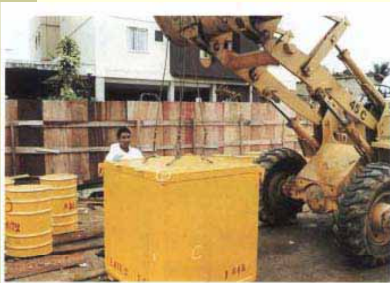
20. One of the specially made 5 tonne waste storage boxes.
