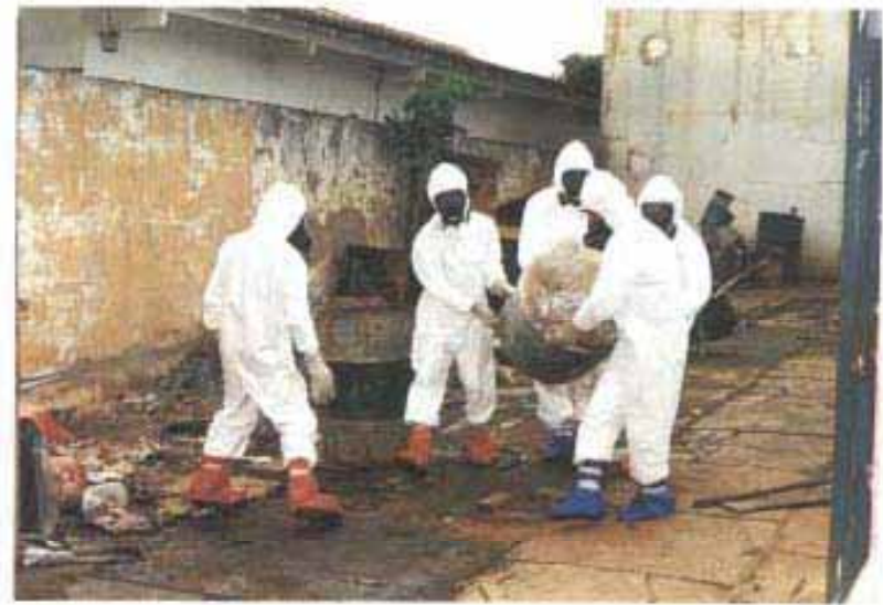
15. Removing contaminated items from Junkyard III.
