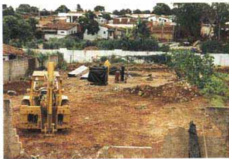
11. Clearing the site at Junkyard II on 6th Street.
