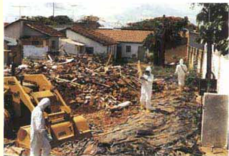
13. Contaminated rubble from the demolition of R.A.'s house on 57th Street.
