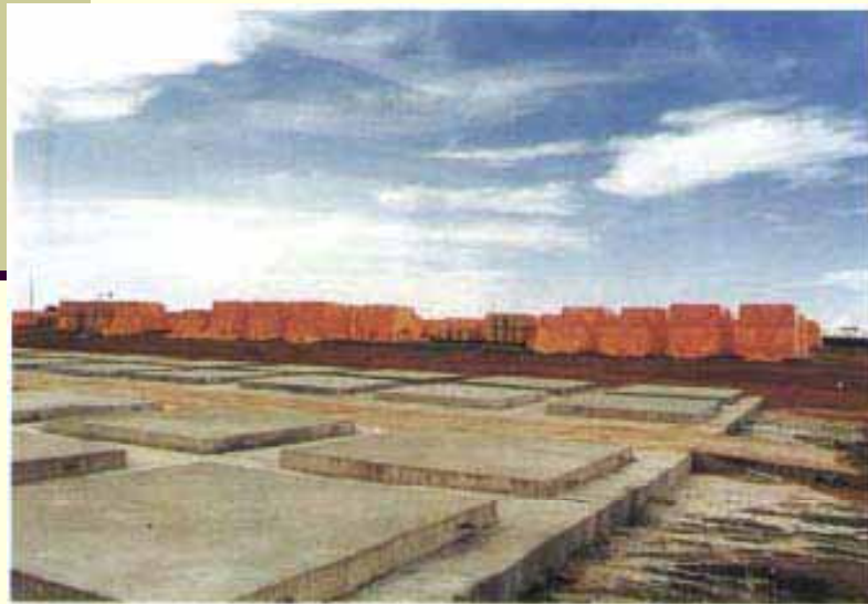
24. The temporary storage site, showing concrete bases with runoff sampling channels.
